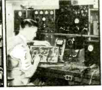
RADIO-ELECTRONIC SERVICE ENGINEER
